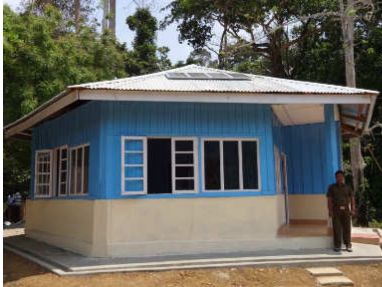
Fig. 23 Inspection Hut at Interview Island (WL) Sanctuary
