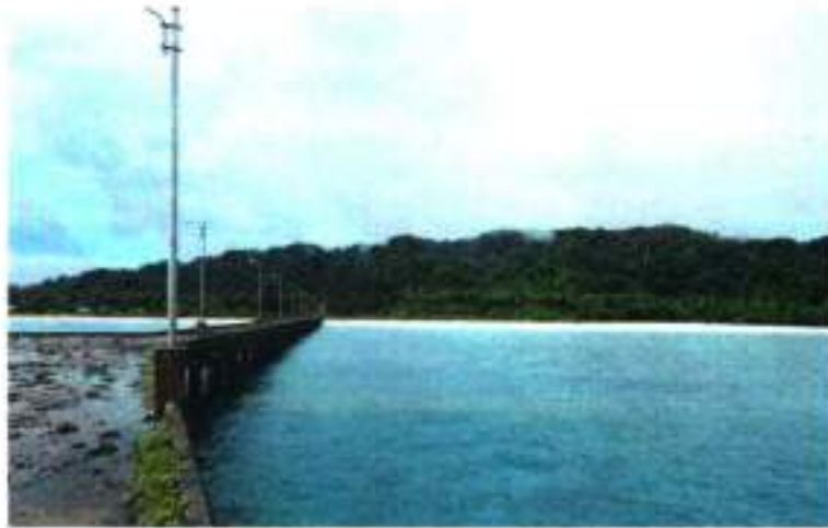
View of jetty at Nemo beach
