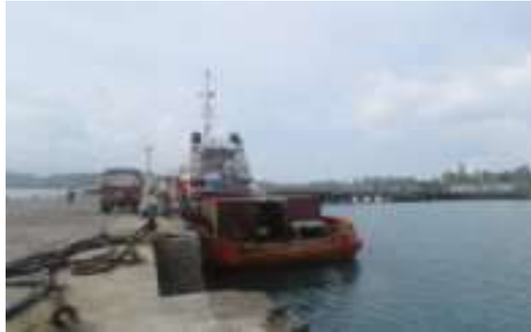
View of jetty at Campbell Bay
