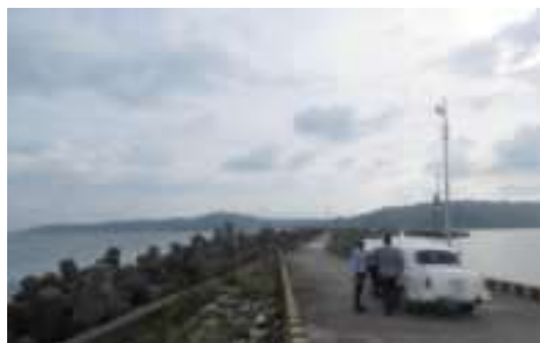
View of breakwater at Campbell Bay
