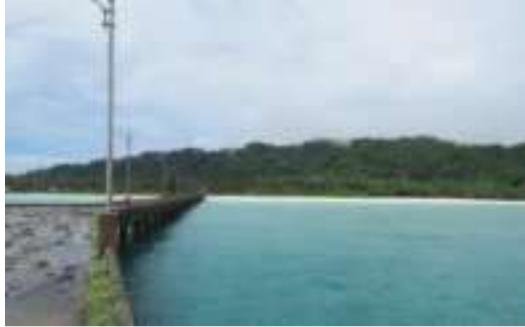
View of jetty at Nemo beach
